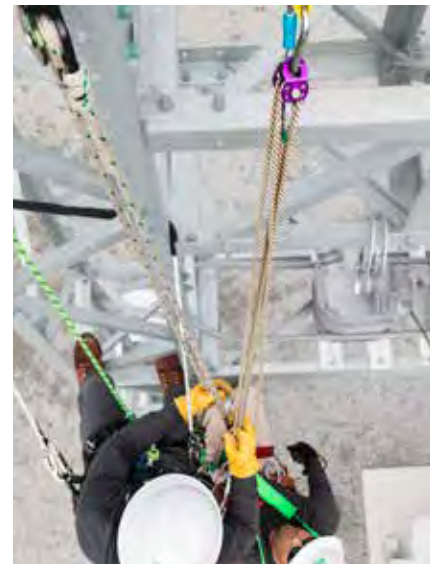
3. Rescue, lowering with the OX BLOCK™.
